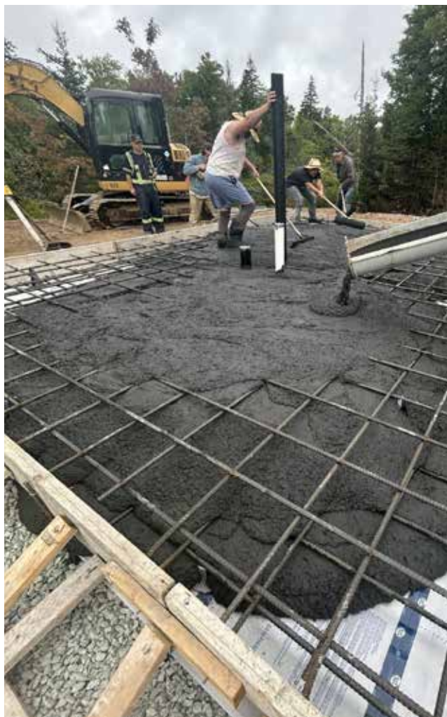
Nova Scotia's Casey Concrete recently demonstrated the cement optimization potential in a slab mix designed with the AlterBiota biochar agent.
